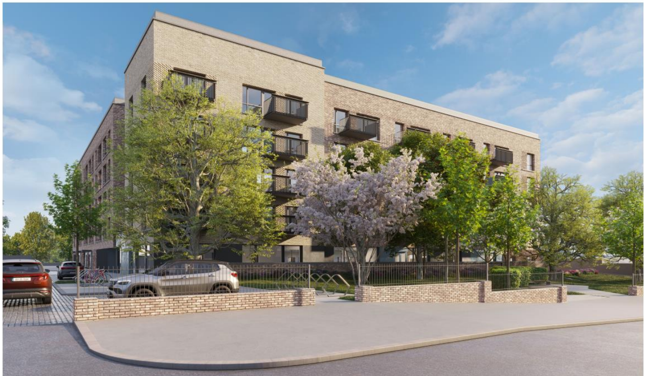
View Looking at the West Elevation onto Cardiffsbridge Road
