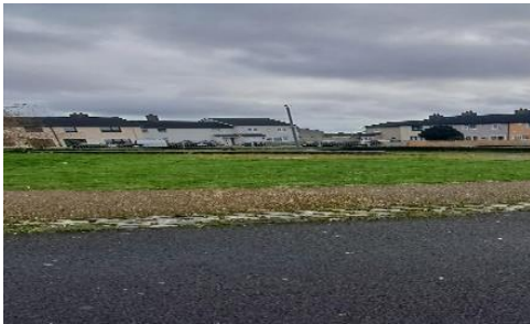
Shangan Park – Before
